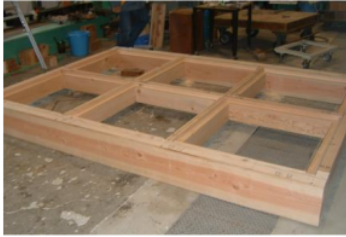
Figure 5. Floor beams system
