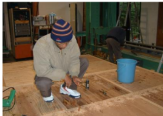
Figure 8. Nailing sugi dowels to panels
