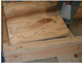
Figure 6. Sheathing floor beams with sugi plywood
