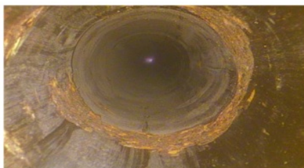
Internal Plastic Coating Condition 2
