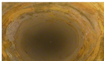
Internal Plastic Coating Condition 3
