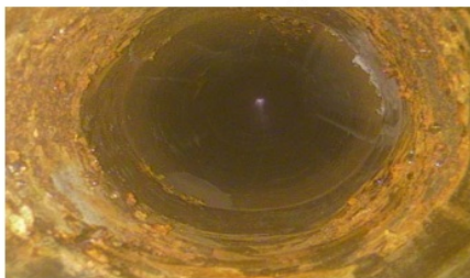
Internal Plastic Coating Condition 4
