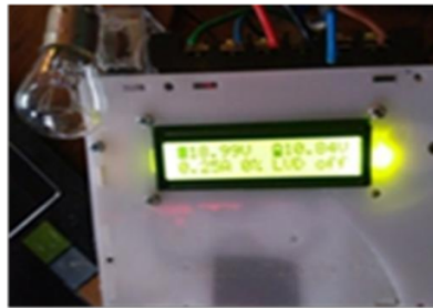
Figure 5. Low Voltage Disconnected condition
