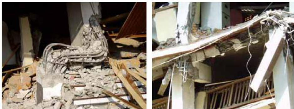
Gambar 2.8. Gempa Yogya 2006, Ground floors soft story (sumber : Boen 2006)
