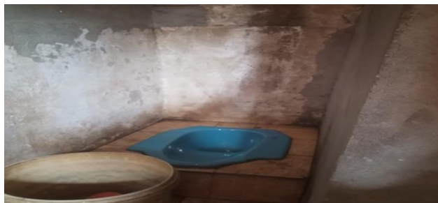
Gambar 4.6 Toilet Pasar Pendopo
