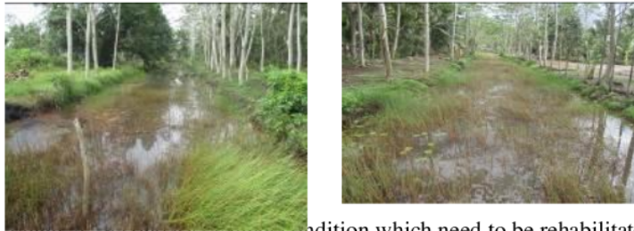
Figure 4. Secondary channel condition which need to be rehabilitated
