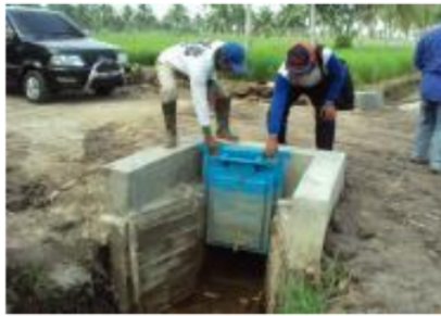
A. Tertiary gate
