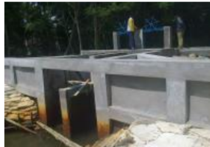
B. Secondary gate
