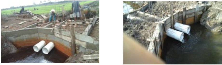
Figure 5. Hydraulic structure in tertiary canal for water retention and control drainage in tidal lowland type C.
