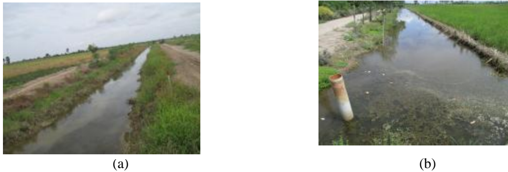
Figure 10. Tertiary channel condition (a) less water at the opened gate and (b) more water due to detention operation
