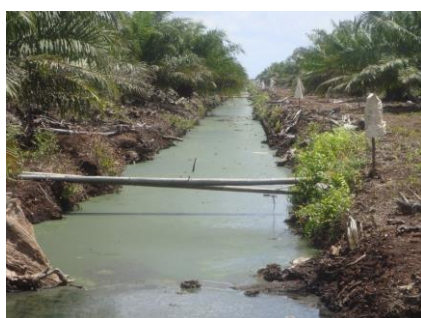
Figure 6. The open channel conditions at tertiary level every 250 m
