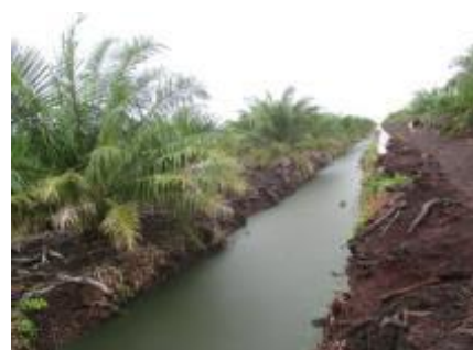
Figure 6. The open channel conditions at tertiary level every 250 m
