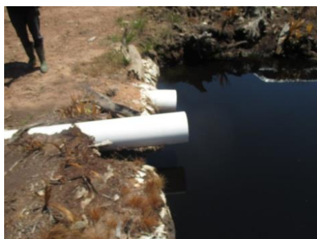
Figure 13. Control of ground water level through water retention in the channel with the water system based on different topography
