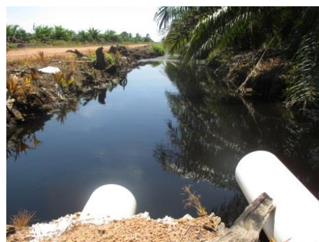
Figure 13. Control of ground water level through water retention in the channel with the water system based on different topography
