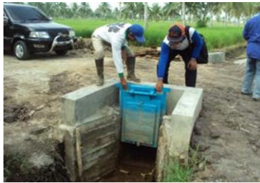
A. Tertiary gate
