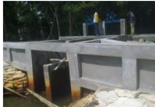
B. Secondary gate
