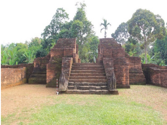
Fig. 7 The door gate of Kedaton Temple made of claystone and quartz arenite
